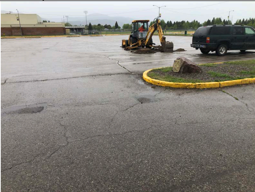
Description: TP-05 Location. View is to the west. Block cracking.
