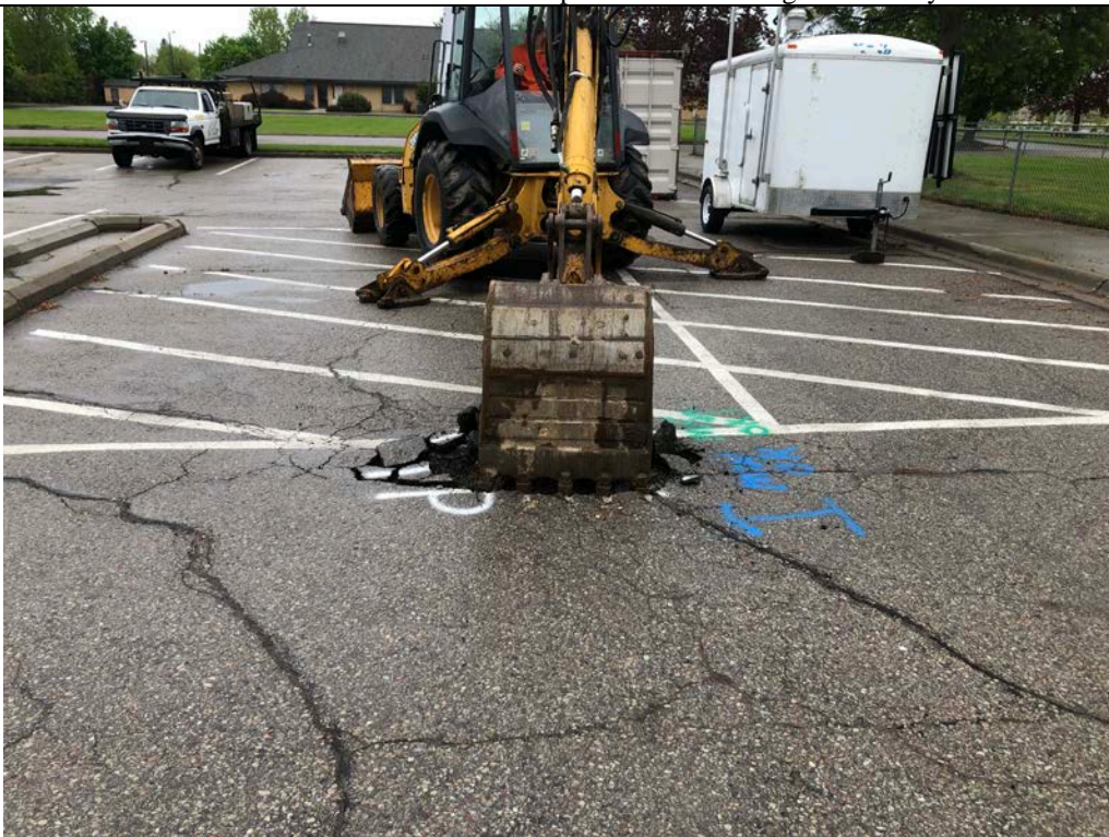
Description: TP-01 Location. Alligator and block cracking.
