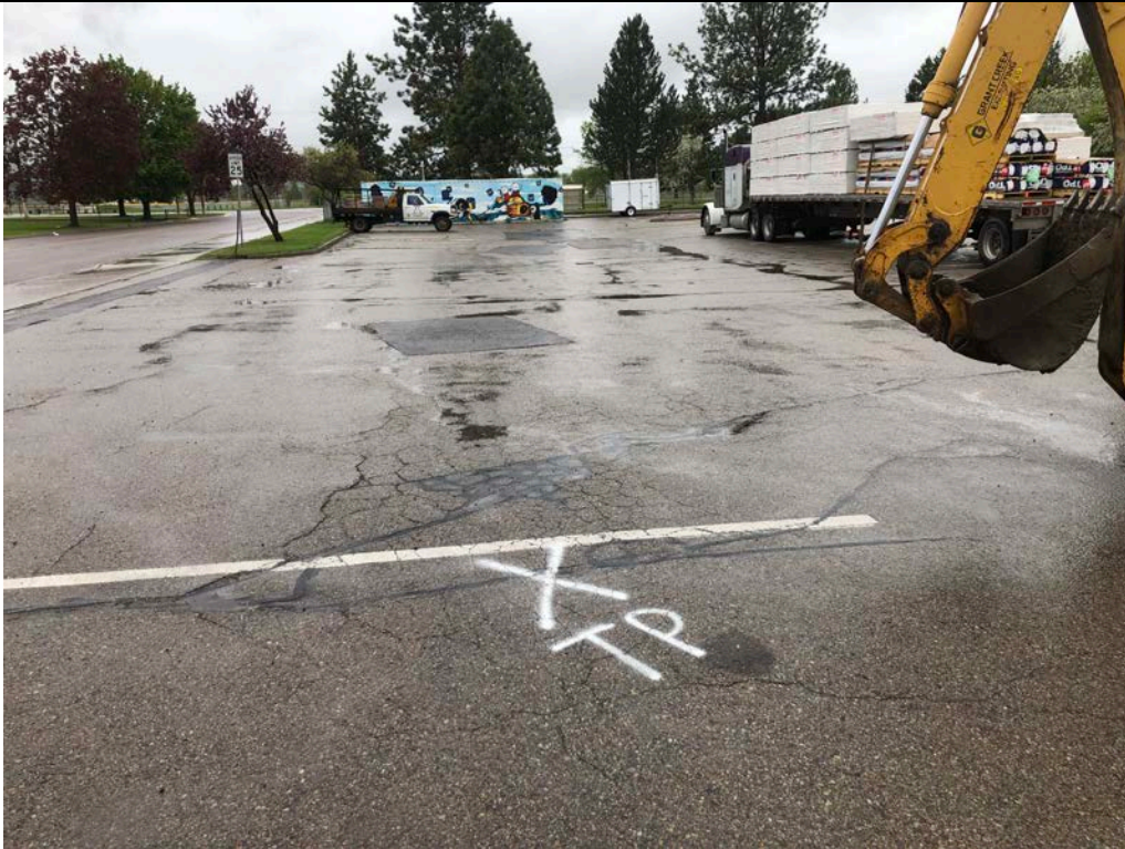
Description: TP-02 Location. Alligator and block cracking. View is to the south.
