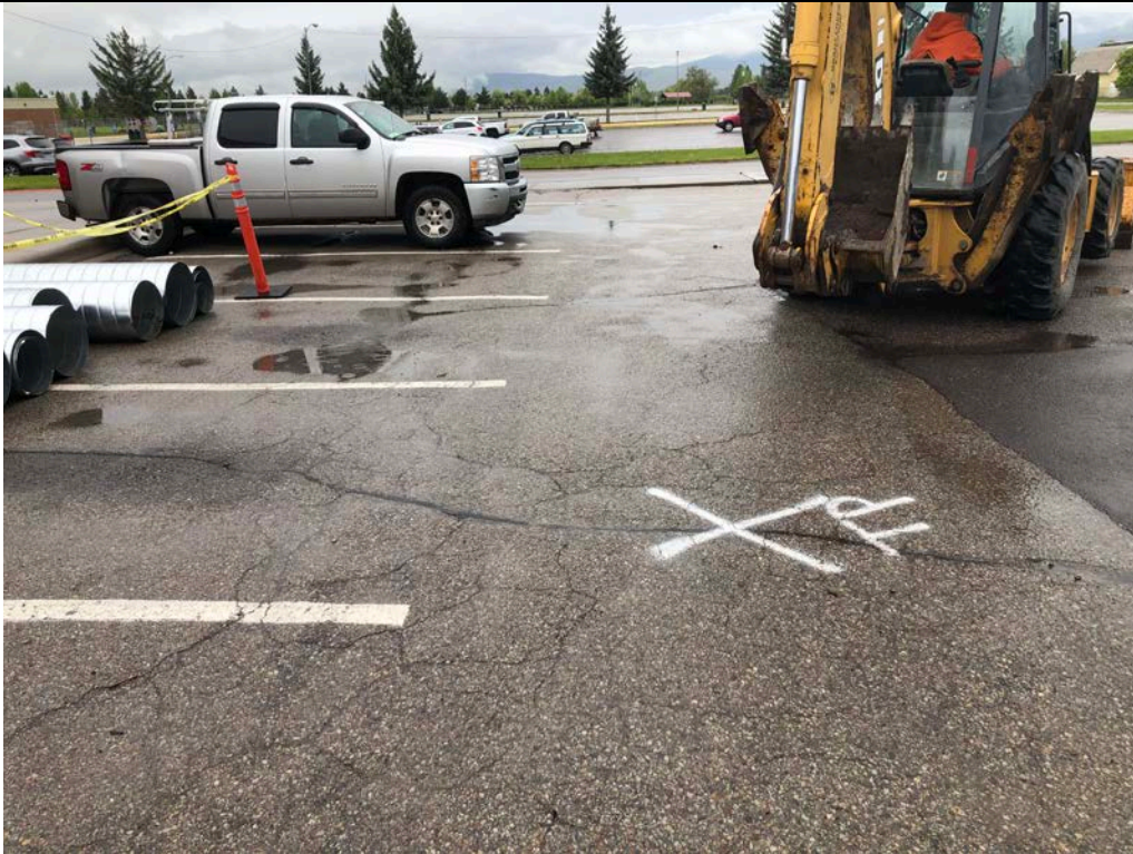
Description: TP-03 Location. Alligator and block cracking. View is to the north.
